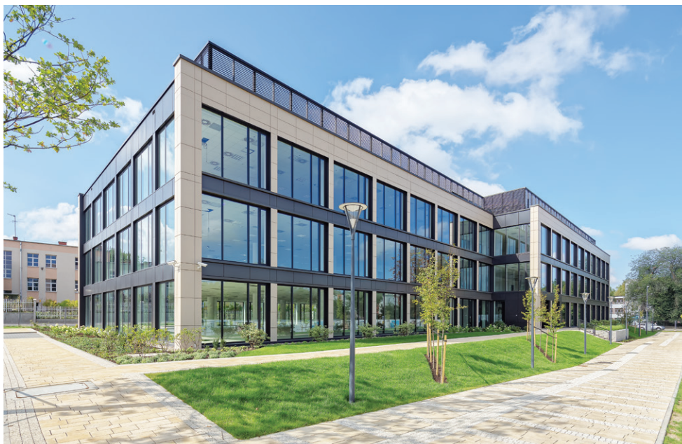
Fot: Radom Office Park
